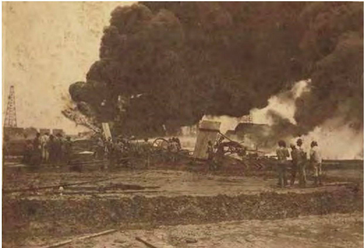
Figure 46. Gas Blowout and Fire at Lake Oil Corp. No. 4 Well at Anse la Butte, Circa 1907. Photograph published by Stickney [2016] from the Special Collections at the University of Louisiana at Lafayette.
