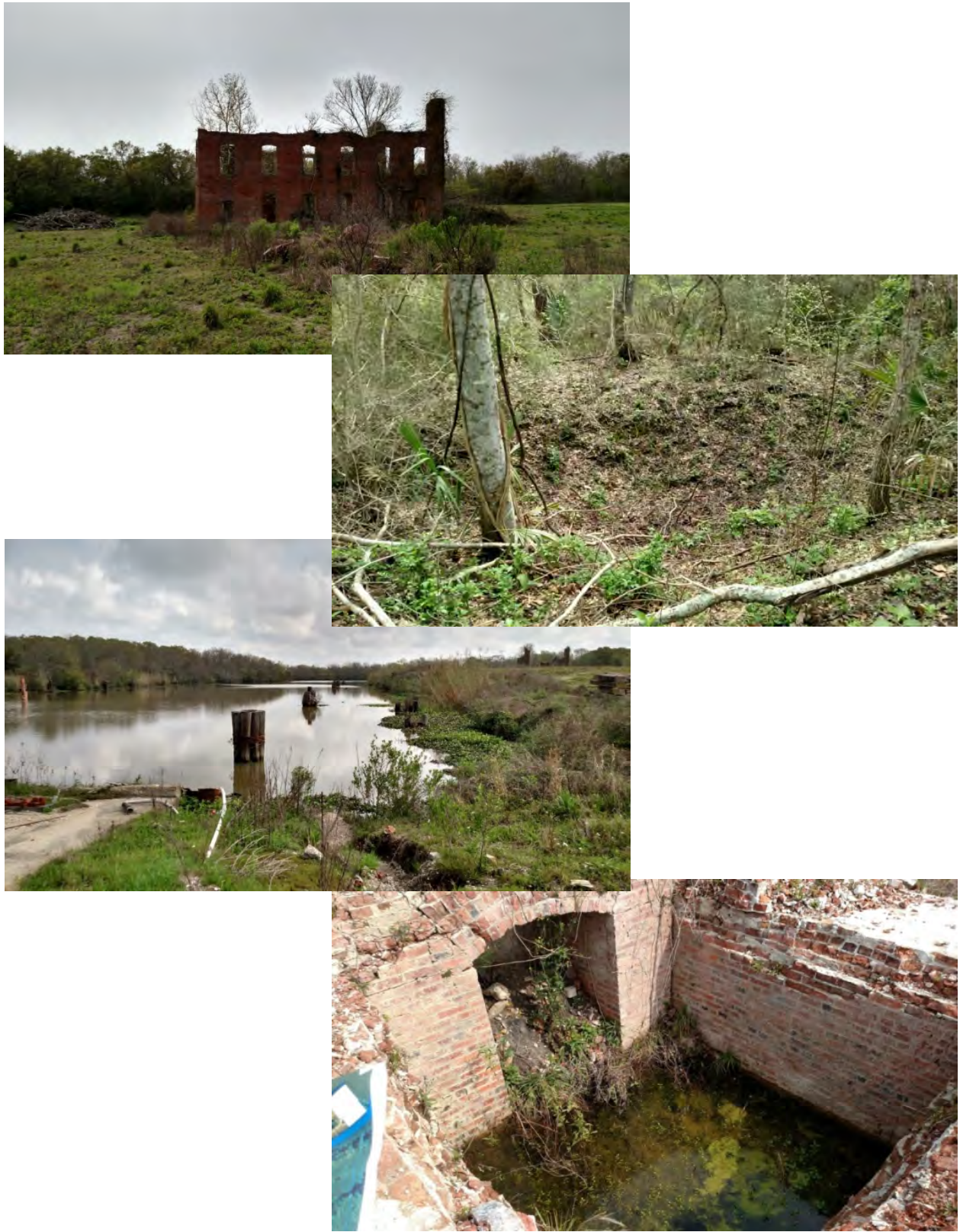
Figure 25. Photographs of the Remains of the Old Belle Isle Salt Mine.
