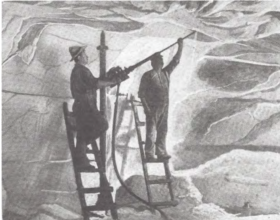
Figure 36. Air Drilling at Weeks Island Salt Mine [Agassiz, 1912].
