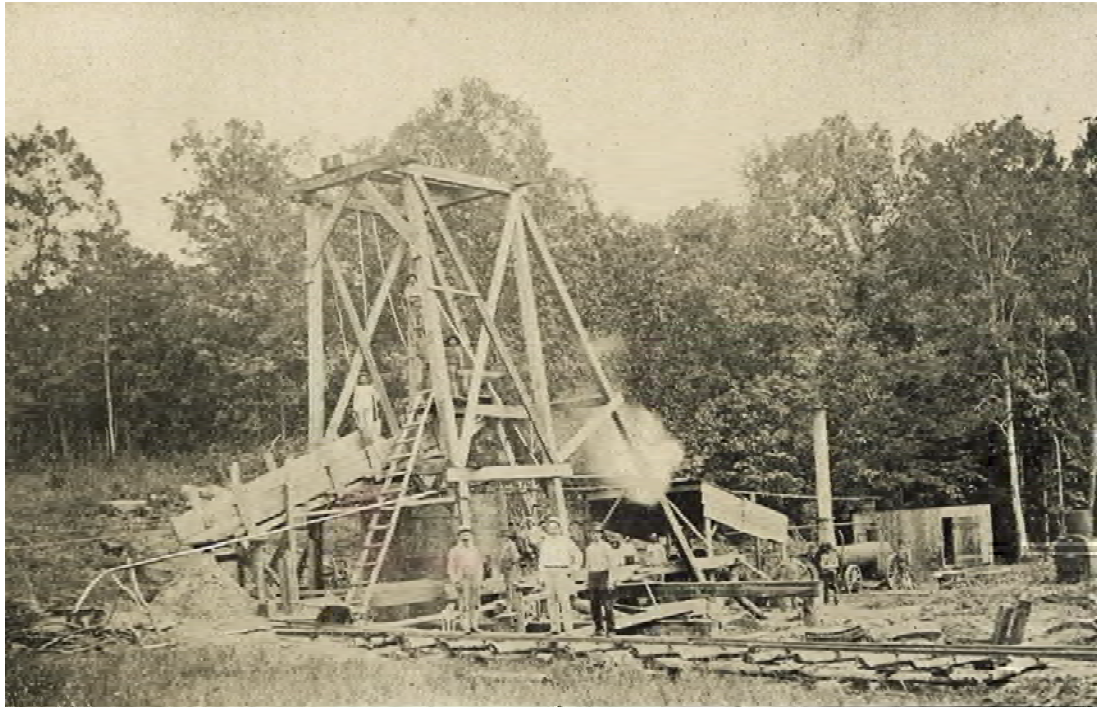
Figure 32. Shaft Sinking at Weeks Island Using Iron Castings from Aborted Calcasieu Sulfur Mine, April 1899. From left to right are G. Cowie (probable), F. F. Myles, and B. B. Myles [Veatch, 1899].
