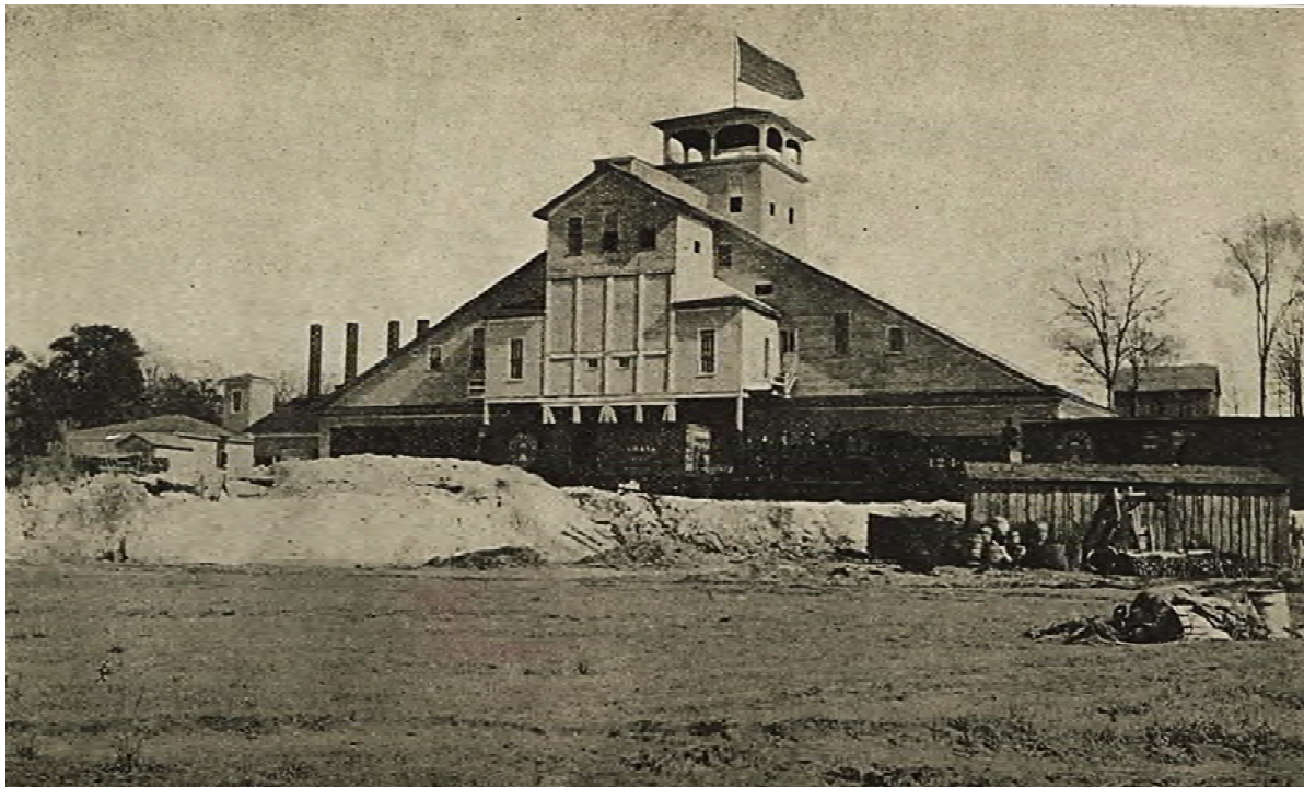
Figure 33. Original Myles Salt Company Mill at Weeks Island That Burned in 1919 [Harris, 1908].
