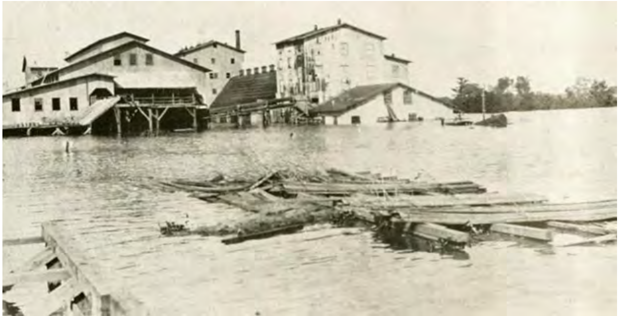
Figure 49. Star Salt Corporation (at Right) and adjacent Baldwin Lumber Company During the Flood of 1927. Water was reported to be 10 feet deep [Louisiana State University, 1927].
