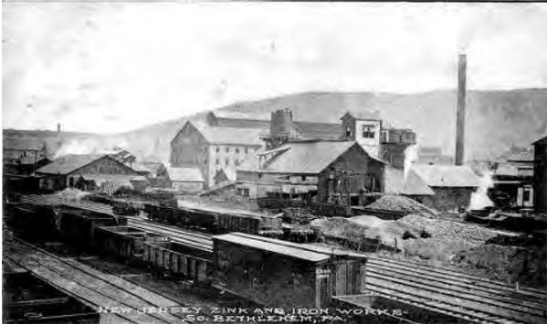
Historic view of the Lehigh Zinc and Iron Company. The Zinc Oxide Works' bag houses are the large buildings at the center of the photo. It was started by Samuel Wetherill. The smoke at the far left is from the Spelter Works started by Joseph Wharton.
