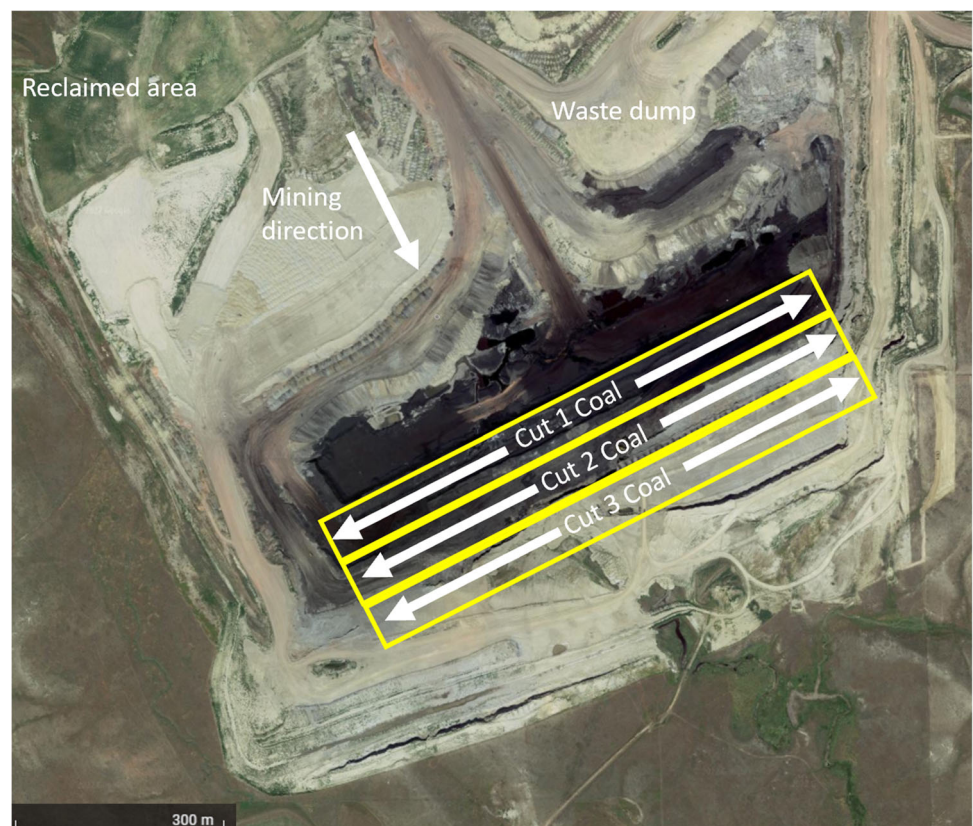
Fig. 11 Example of truck and shovel mine layout from a PRB mine showing mining benches, contemporaneous reclamation, waste dumps, and mining direction. Adapted from: [49] Photo by: [51]
