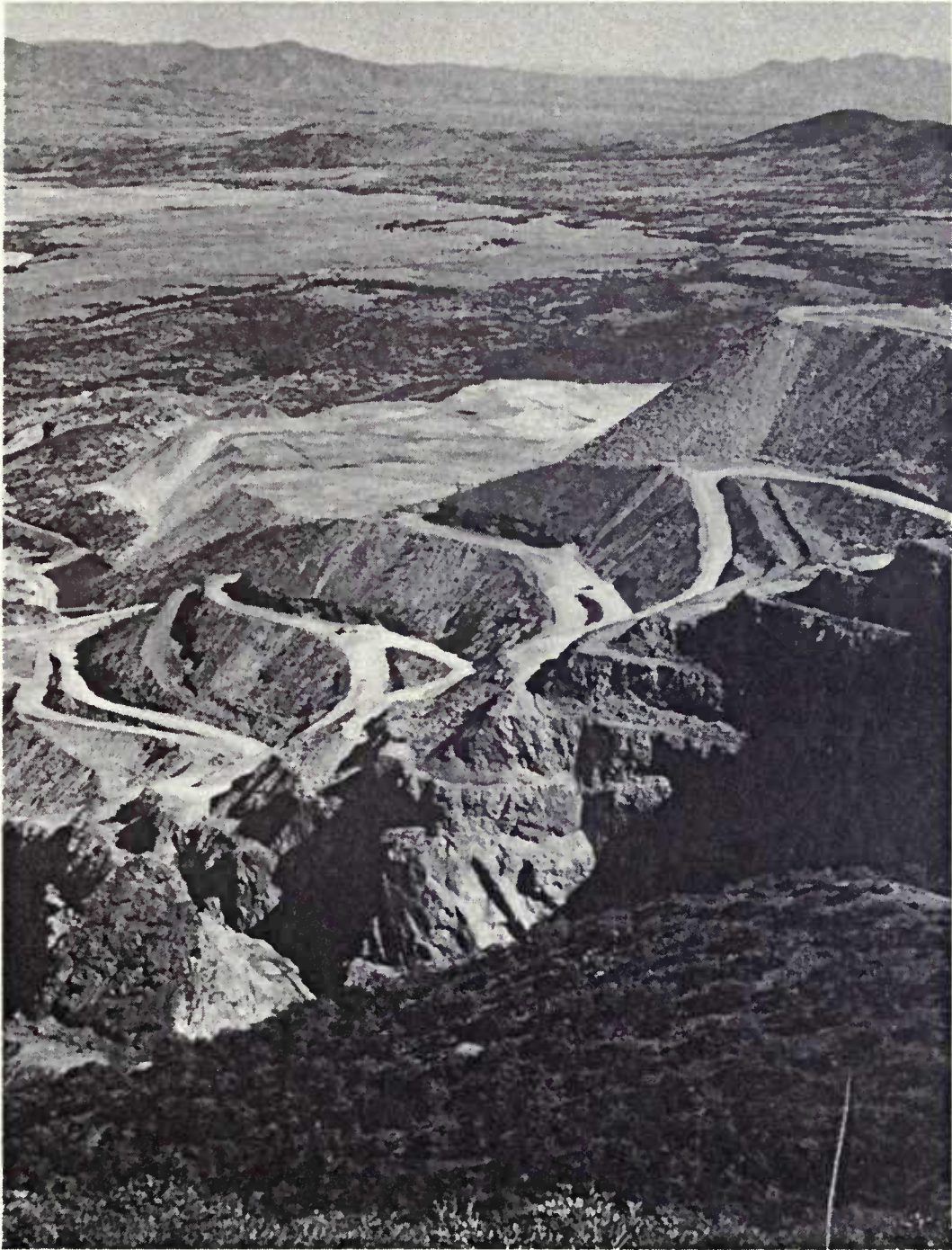
La Colorada open pit, Cananea, Sonora, Mexico. Looking easterly, the Ajo Mountains in the background. March 1973. The picture illustrates the steep mining slopes maintained in the open pit because of the unusual hardness of the rock.
