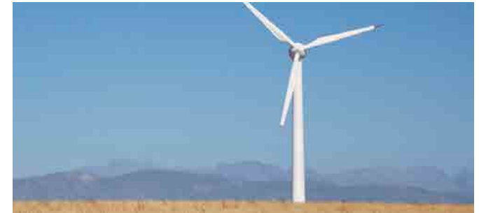
Windturbine - Renewable Energy
