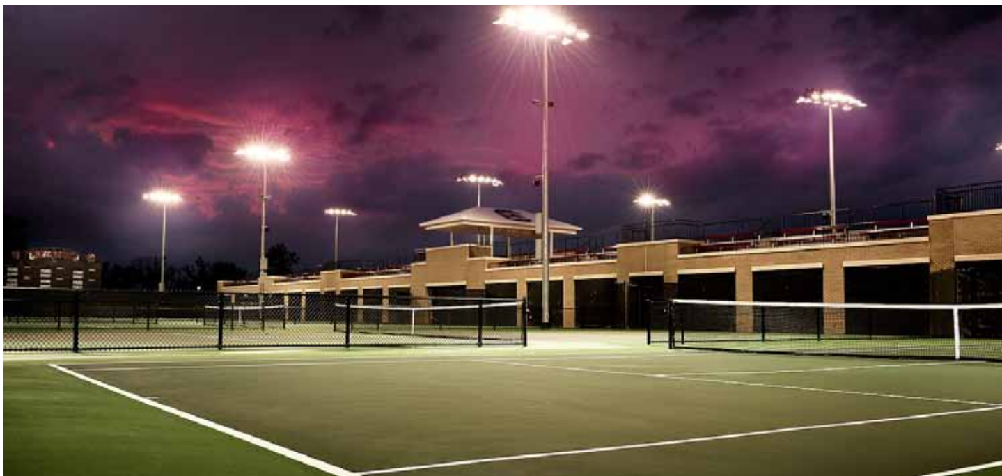
The spring of 2012 marks a new era for South Carolina tennis as the Gamecocks open a $4.6 million facility that will accommodate both men's and women's programs. Located in the heart of the Athletics Village at the Roost, the stadium features 12 courts with lights and scoreboards on each one. Each side of six courts also has a master scoreboard so fans always know what's happening on each court. Video cameras are mounted behind each court as well to record matches and stream them live over the internet. Seating is available for 670 fans with plenty of standing room available for more. The stadium has 400 square feet of court-side storage and 900 square feet of dedicated restroom facilities.
