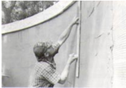
Air entraining and plasticizing ease application and reduce shrinkage.
