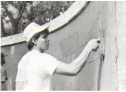
Air entraining and plasticizing ease application and reduce shrinkage.
