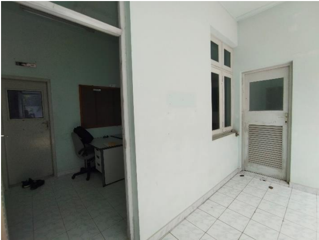
Image 6: SME Hub Building A (Kiosk)
