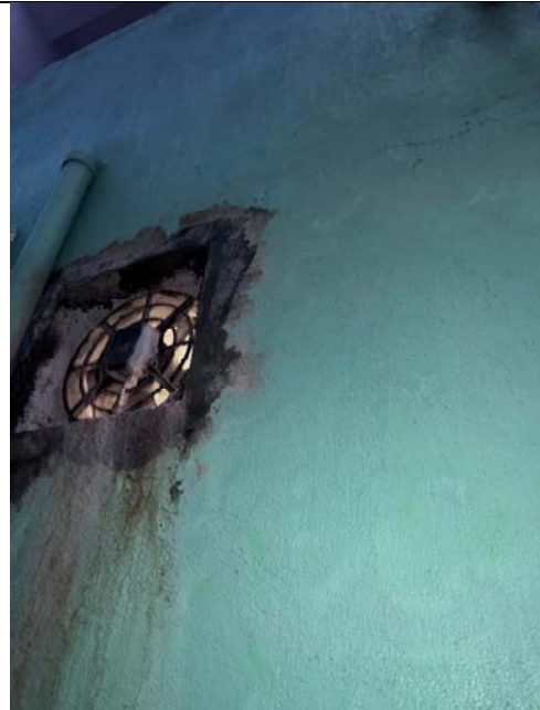
Water leakage to exterior wall from an internal wall pipe
