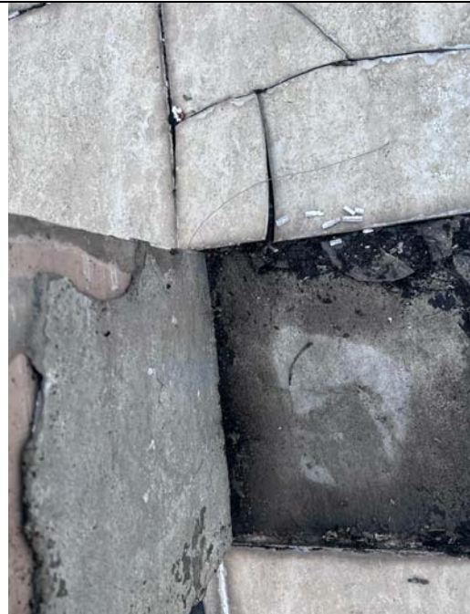
Water leakage to exterior wall from an internal wall pipe
