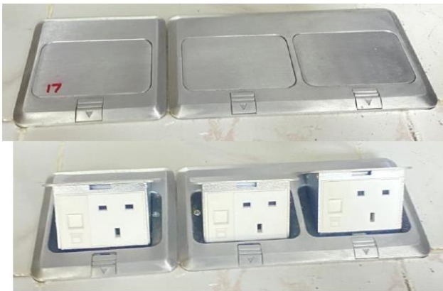
Floor Socket with RG45 network face plate
