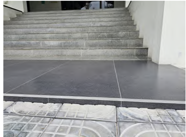
Required standards for the finished tiling work
