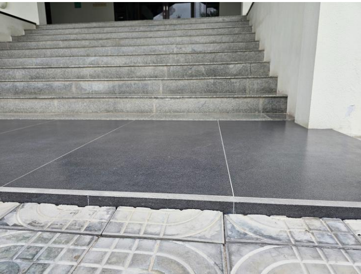
Required standards for the finished tiling work
