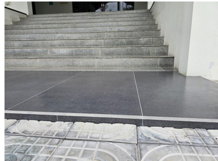
Required standards for the finished tiling work
