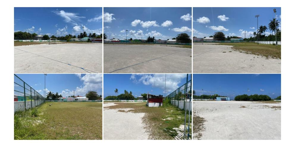
Ground Conditions: Proposed site is located due North / East side of the island;4 trail holes were made. Noticed +/- 300 mm of soil (generally fine and soft) have to be removed and back filled, it was noticed that the plot is slightly lower than existing main road.
