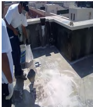
Fig 2. Broad casting Quartz for Mechanical Key
