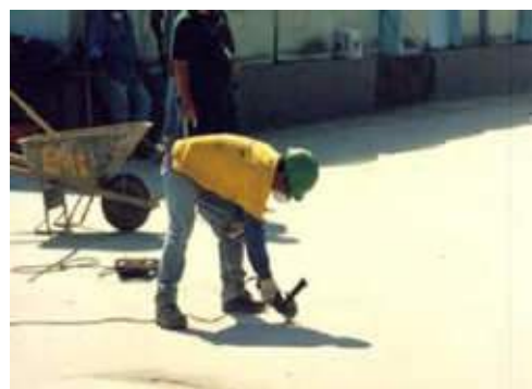
Fig 2. Determine and chasing the cracks
