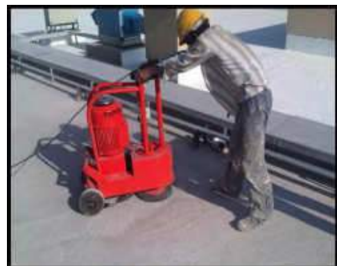
Fig: 2 Preparations with Grinder
