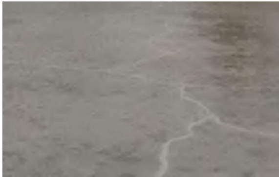
Fig Cracks filled with Epoxy Mortar
