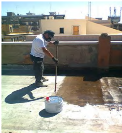
Fig 1. Priming the Surface
