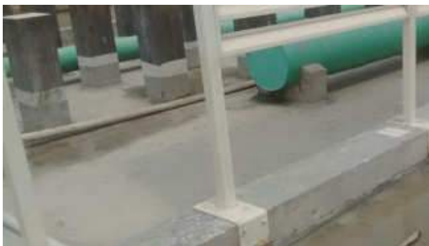
Fig 1 . Coving of the joints and Up stand
