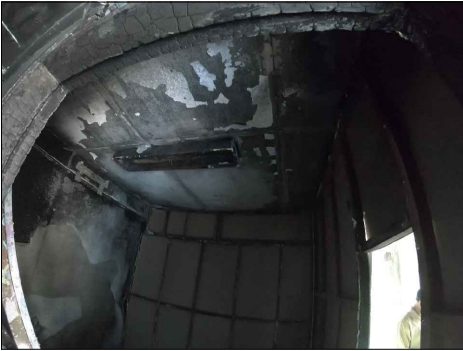
Re-plaster and fix all burnt walls
