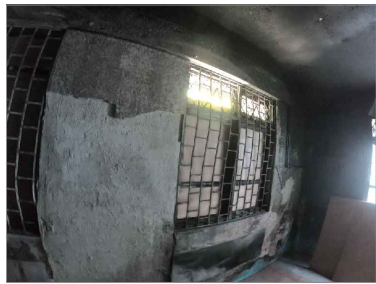
Re-plaster and fix all burnt walls
