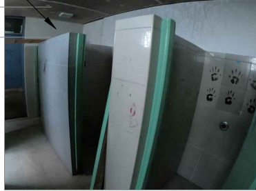
Re-plaster and fix all burnt walls
