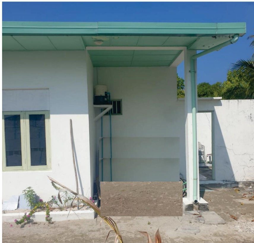
New toilet area
