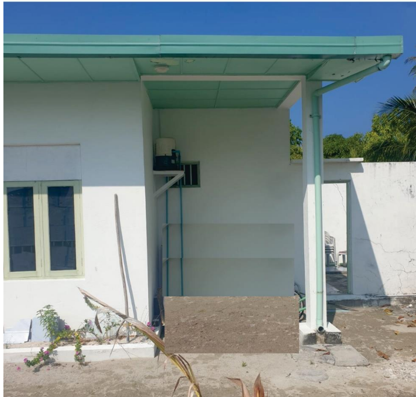
New toilet area
