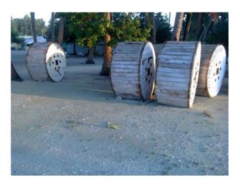
(Outer cover of cable drum must be properly packed and covered)
