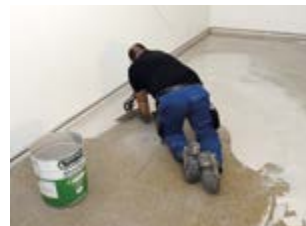
Application of main coat
