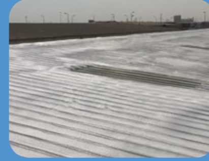
INSULATED STEEL ROOF WITH WATER PROOF SYSTEM
