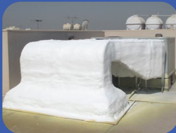
INSULATED AC DUCT
