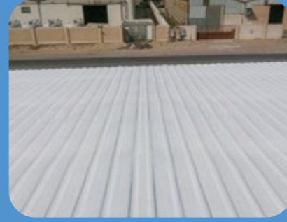
INSULATED STEEL ROOF WITH WATER PROOF SYSTEM
