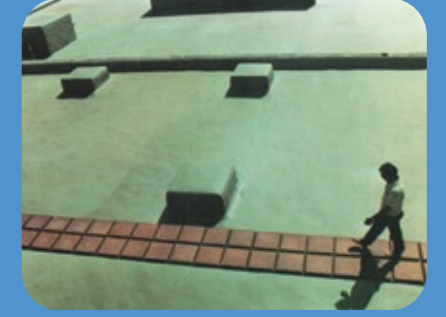
FINISHED ROOF WITH PAVER WALKWAY
