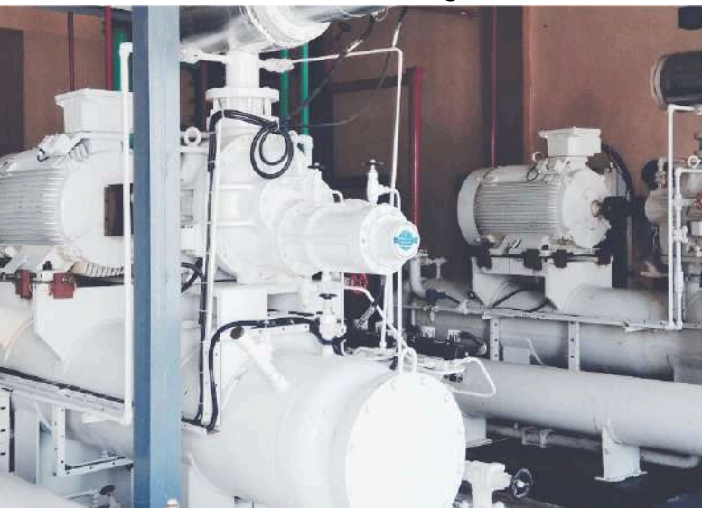
1 Ton/Hr IQF at -45 Deg C, 2 Nos. 750 Kg/hr. Plate Freezers at (-)40°C, 120 Tons Flake Ice Machine with 2500 Ltr/hr. water chillers
