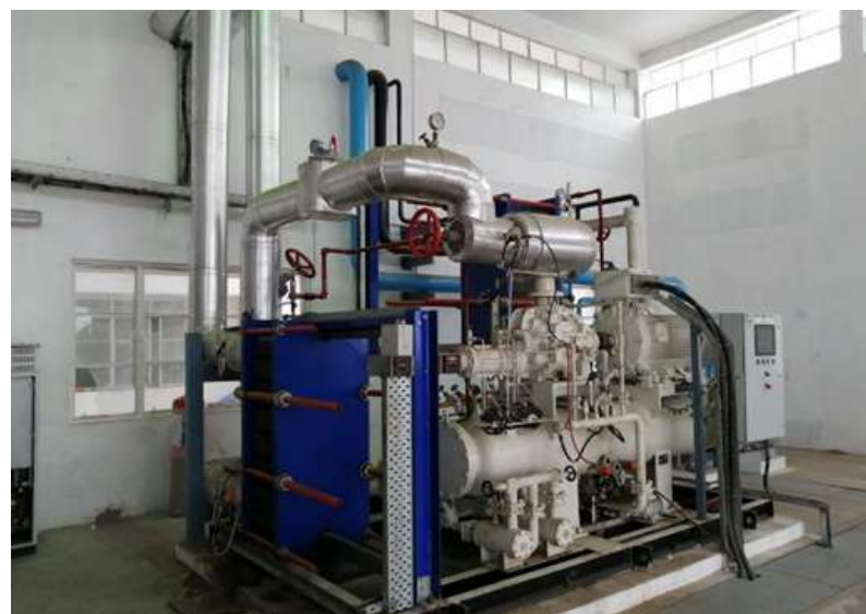
2000 TR (7000 kW) ammonia refrigeration system for chilled water cold rooms (various application (-)10, (-)5, (-)2 and (-)15°C)
