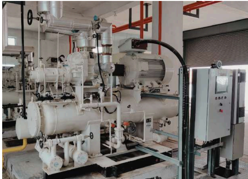
Methanol Chilling Plant 20 TR of Methanol Chilling at (-)55°C
