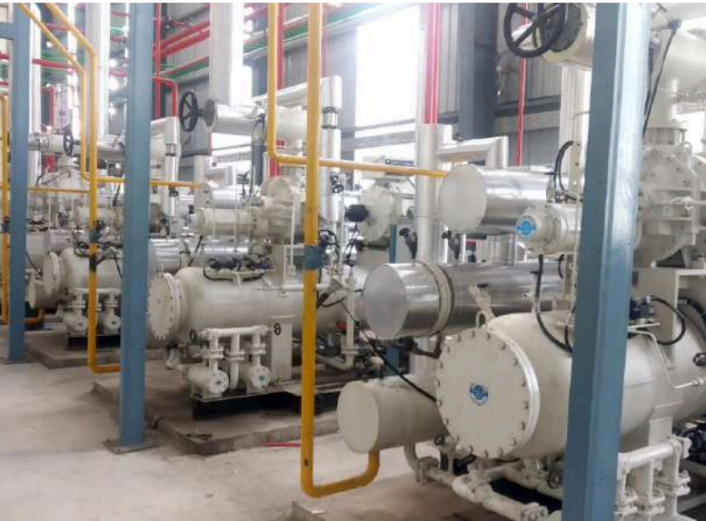
10 TR of TUNA Freezing plant at (-)65°C with ammonia as Refrigerant
