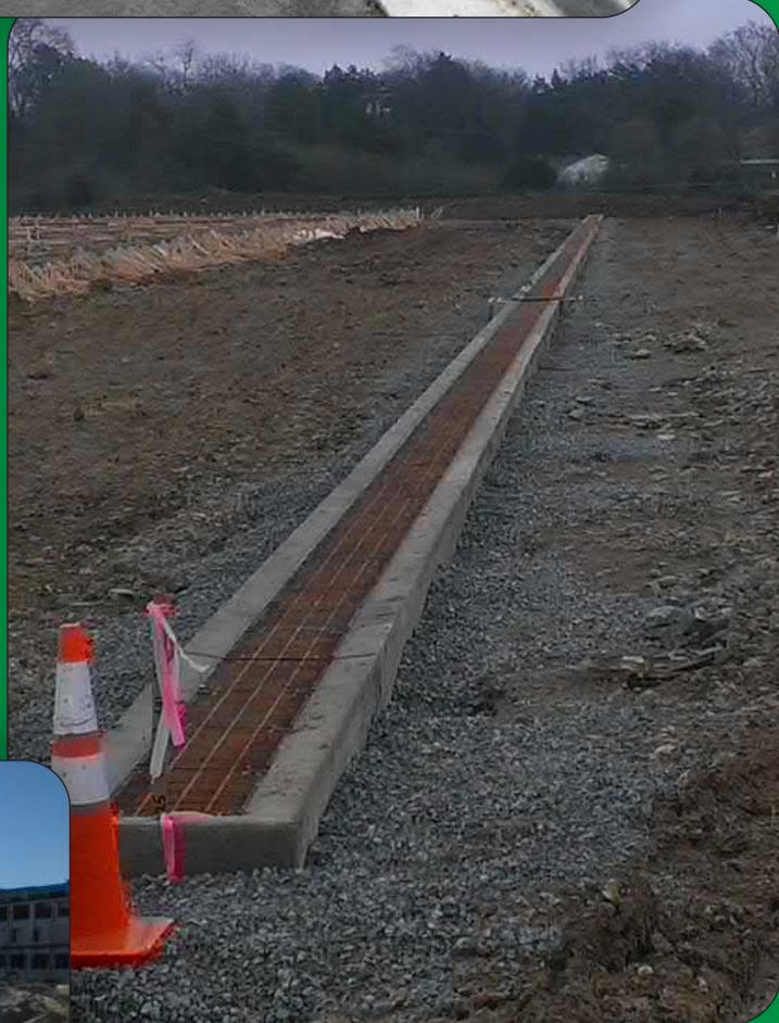
Concrete formed trenches are generally more expensive to construct due to the lack of skilled labor and wage rates. With the Dura Trench prefabricated forming system much of this labor and skill is removed. The end results look basically the same as a prefabricated trench from the surface, but in some instances are preferred to a prefabricated trench. No matter what system you need, Dura Trench has a solution for your linear drain needs.
