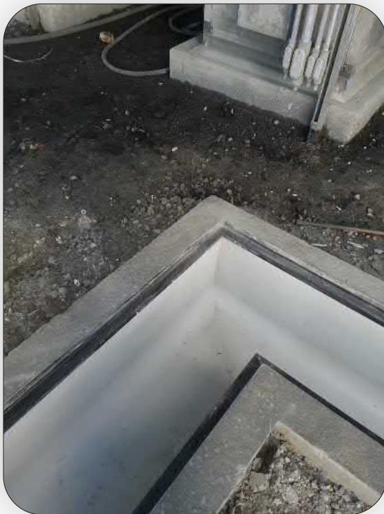
Factory built turns, intersections, and unique fabrications are important advantages of the Dura-Trench line. These shop made fabrications ensure a high quality connection and a good fit. Prefabricated parts save significant time in the field making the Dura-Trench system the easiest product on the market to install.
