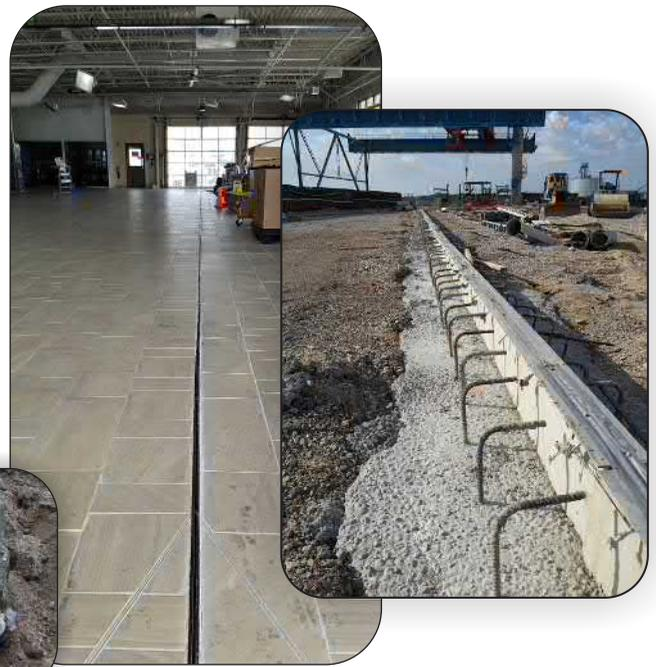
Slotted drains typically outlet with a pipe out the end or by using a catch basin. The Dura-Trench system is offered with any size outlet pipe connection desired, molded directly into the system for easy field connection to the drainage piping system.
