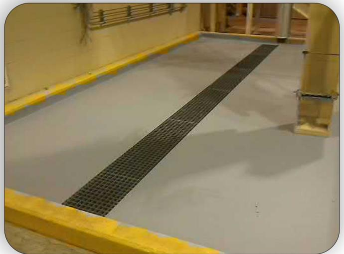
Chemical trenches are available with 100% composite construction with no metal components. With certain chemical combinations even stainless steel materials can be compromised. In these applications a 100% polymer trench can be a viable solution.
