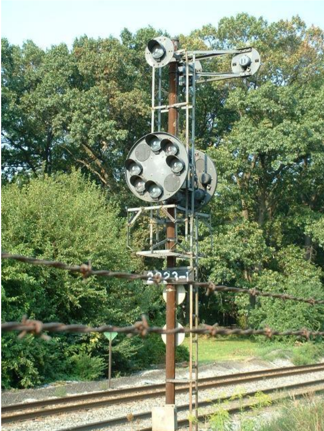
Both sides of the same CPL location at the Gaithersburg fairgrounds in suburban Washington DC. Both tracks are signaled thru here for bi-directional operation.
