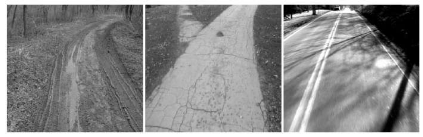
single-lane dirt access road
