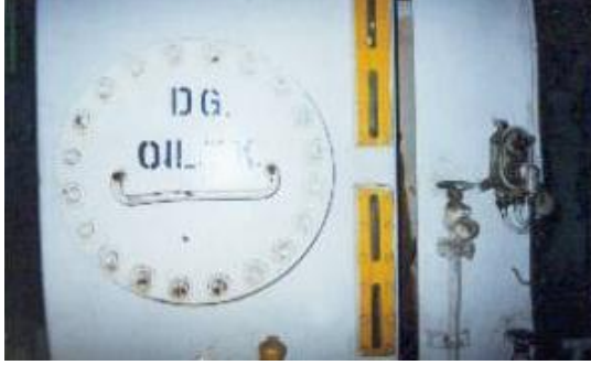
D.G Oil tank
