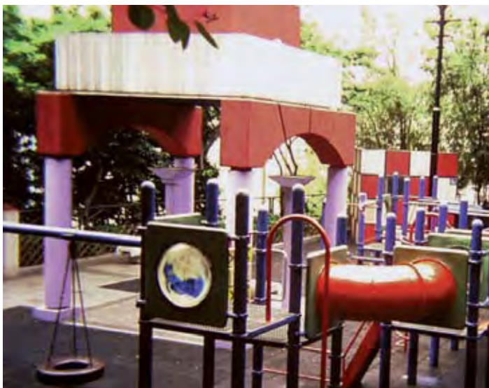
Fig. 11.16 Hard surface. This attractive play area for children has a serious flaw: a concrete surface. The children may stay cleaner but are much more likely to sustain injuries with falls.
