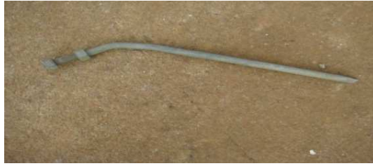
Gambar 56 Penghalang panjang / ACD ( Anti Climbing Device )
