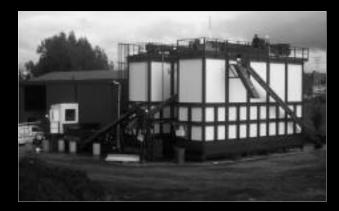
A vertical closed vessel compost unit in Waitakere, New Zealand. Waitakere is town of 80,000 households within the Aukland region. The unit has a capacity of 14,000 tonnes a year, using ten chambers, which allows different qualities of feedstock to be processed separately.
