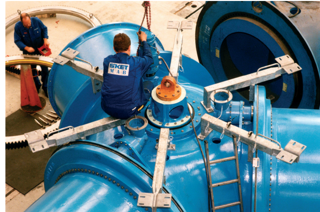
Figure 8.1 SKET wind turbine production
