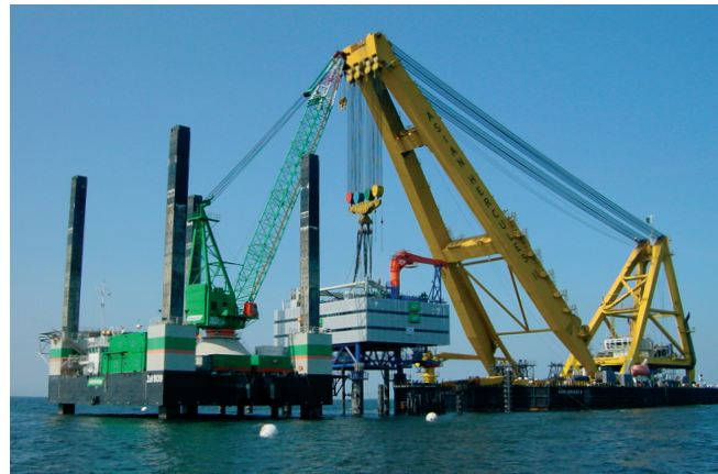
Figure 5.5 Installation of HornsRev transformer
