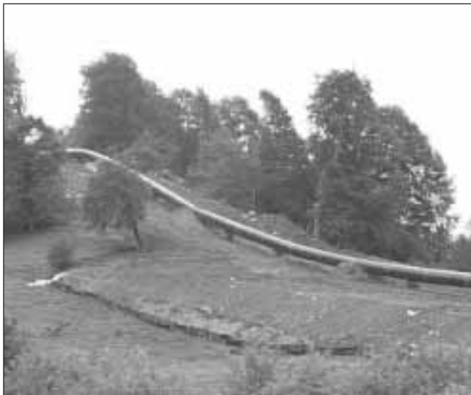
BTC pipeline construction in the Borjomi National Park, Georgia, 2004 (WWF).
