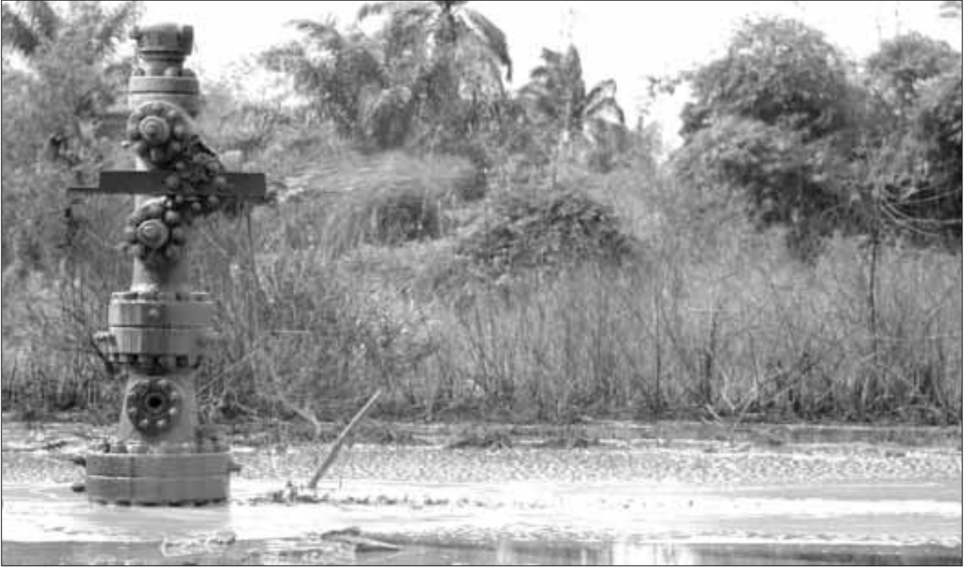
Leaking oil 'Well-Head 18' in Kpor, Ogoni, Nigeria [2004]. The crude oil is turned brown when mixed under the high pressure with the natural gas also being carried in the pipes. Local witnesses reported that the oil well, that is part of Shell reserves, had been leaking at this rate for five months. Local streams and wells for drinking water were heavily polluted with crude oil. According to the local 'Chief of Compound' this was the third spill since 1959 (© Tim Nunn/SDN).
