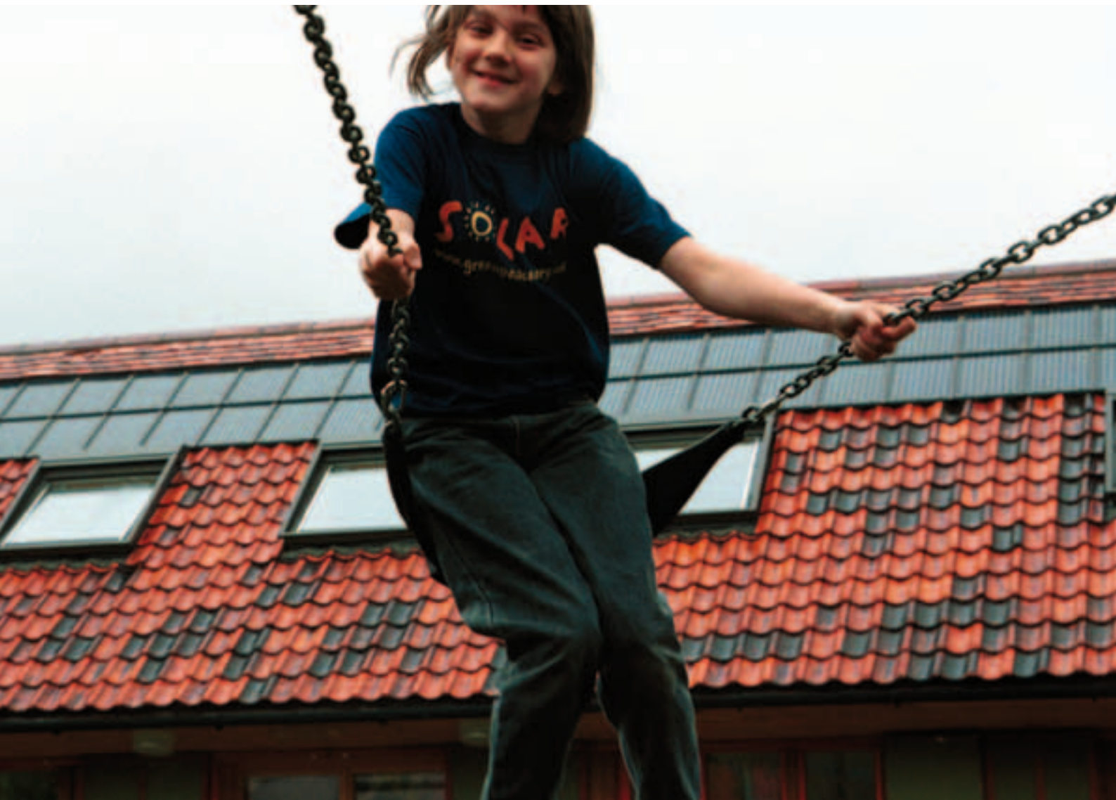
Photovoltaic installation at an inner city playground, London. ©Greenpeace/Davison.
