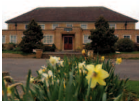
South Somerset District Council plans to install a 50kw wind turbine at this school to reduce the school's energy bill by £7,000 per year. ©SWNS.
