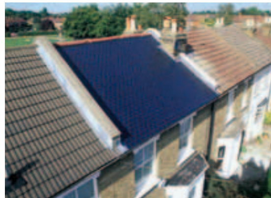
Jeremy Leggett of Solar Century was one of the first to fit his home with building integrated photovoltaics.
