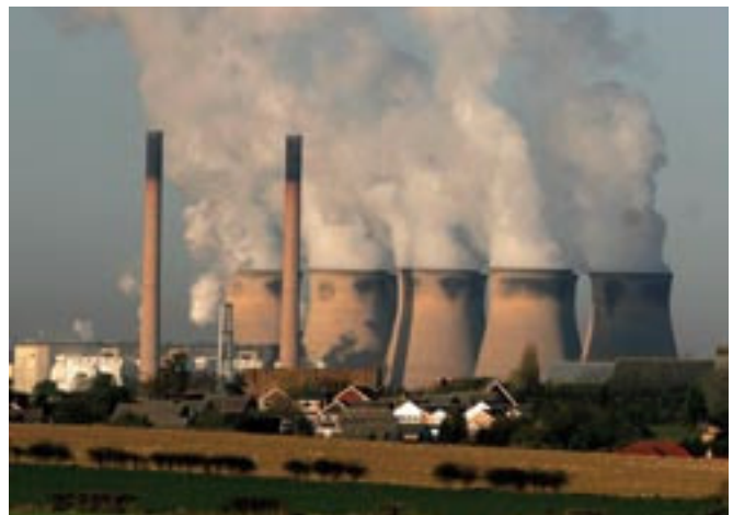
Large power stations far from cities waste two-thirds of the energy generated through their cooling towers – equivalent to the total heat demand (eg heating, hot water) of all buildings in the UK. ©Greenpeace/Morgan
