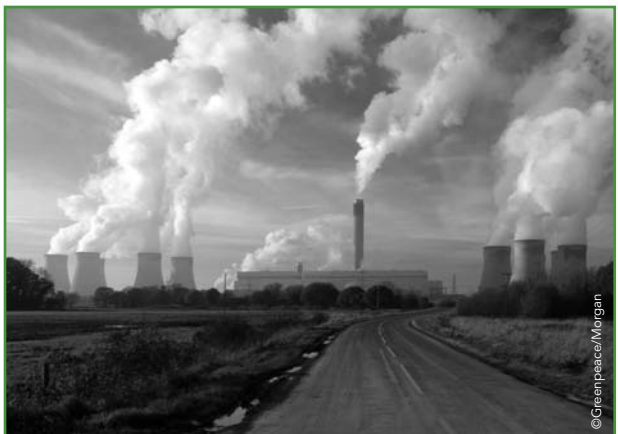
The Drax coal power station typifies the problems of centralised system – most of the energy is lost as heat up the cooling towers.
