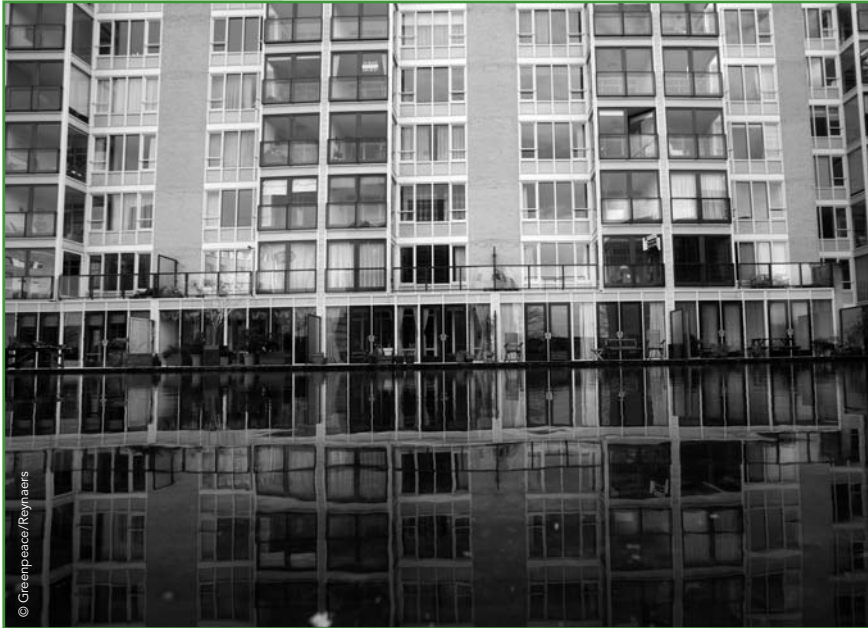
This housing development in Amsterdam gets its heat and power from a community CHP plant.
