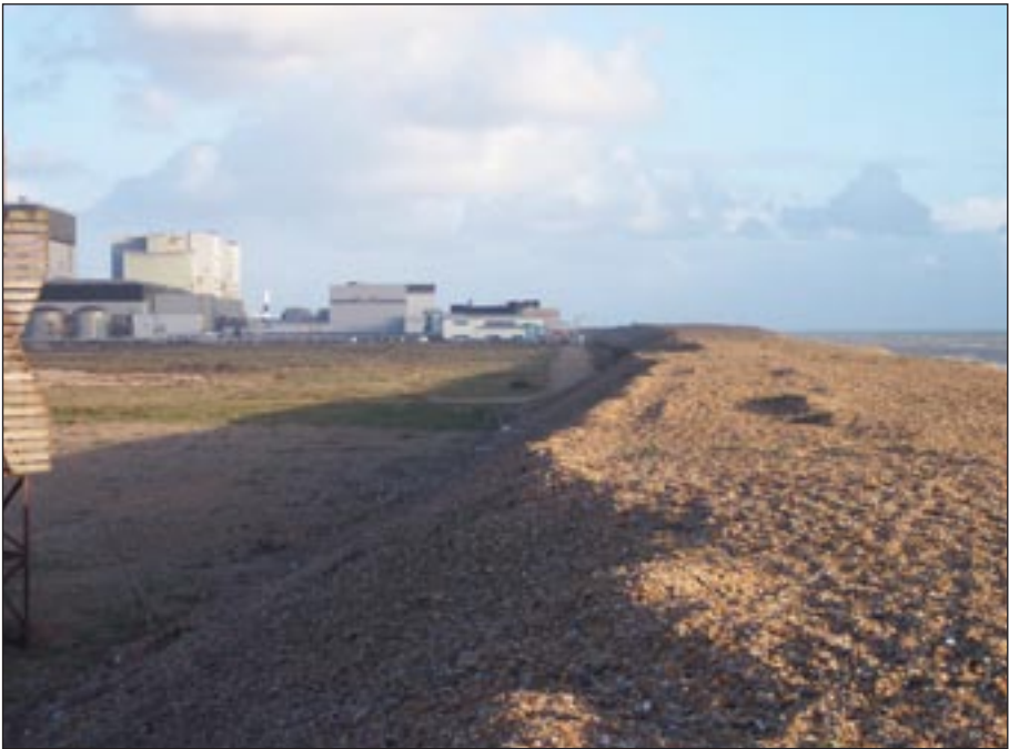
Photo 1. Profiling of the gravel ridge at the nose of the foreland attempts to safeguard the power stations. However, with increasing storm surge heights, re-profiling may result in over-steepening. This increases the susceptibility to barrier breakdown and breaching, which would result in widespread flooding of the area.
