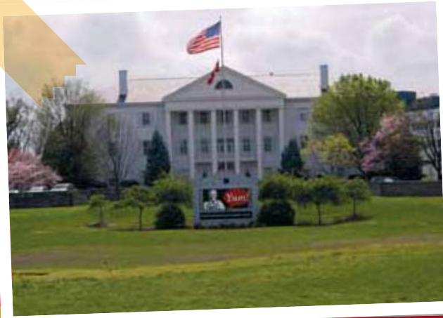
Yum! Brands and KFC International head office, Louisville, Kentucky, USA.
