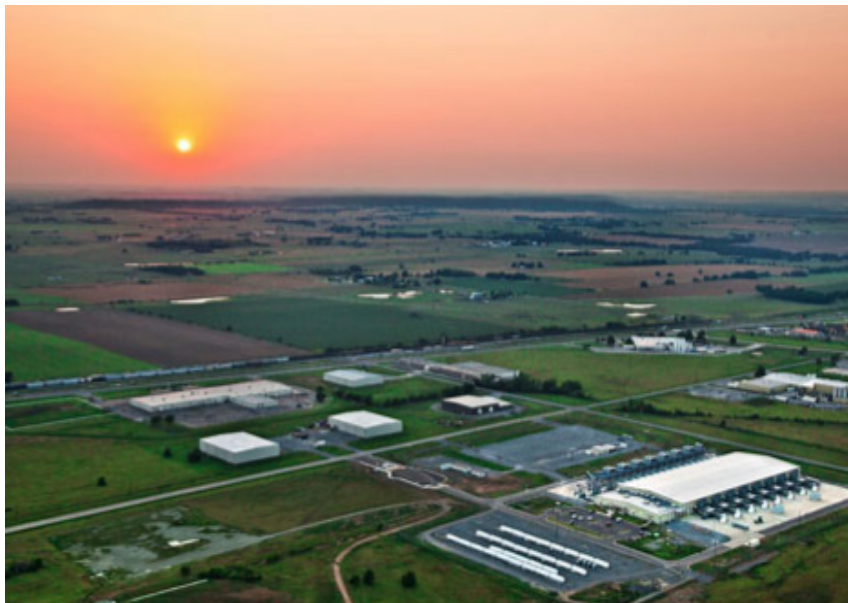
Google Oklahoma data center campus
