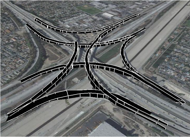
Figure 6: Successful reconstruction of multiple overlapping overpasses of the I-105/I-710 Interchange in Compton, California.
