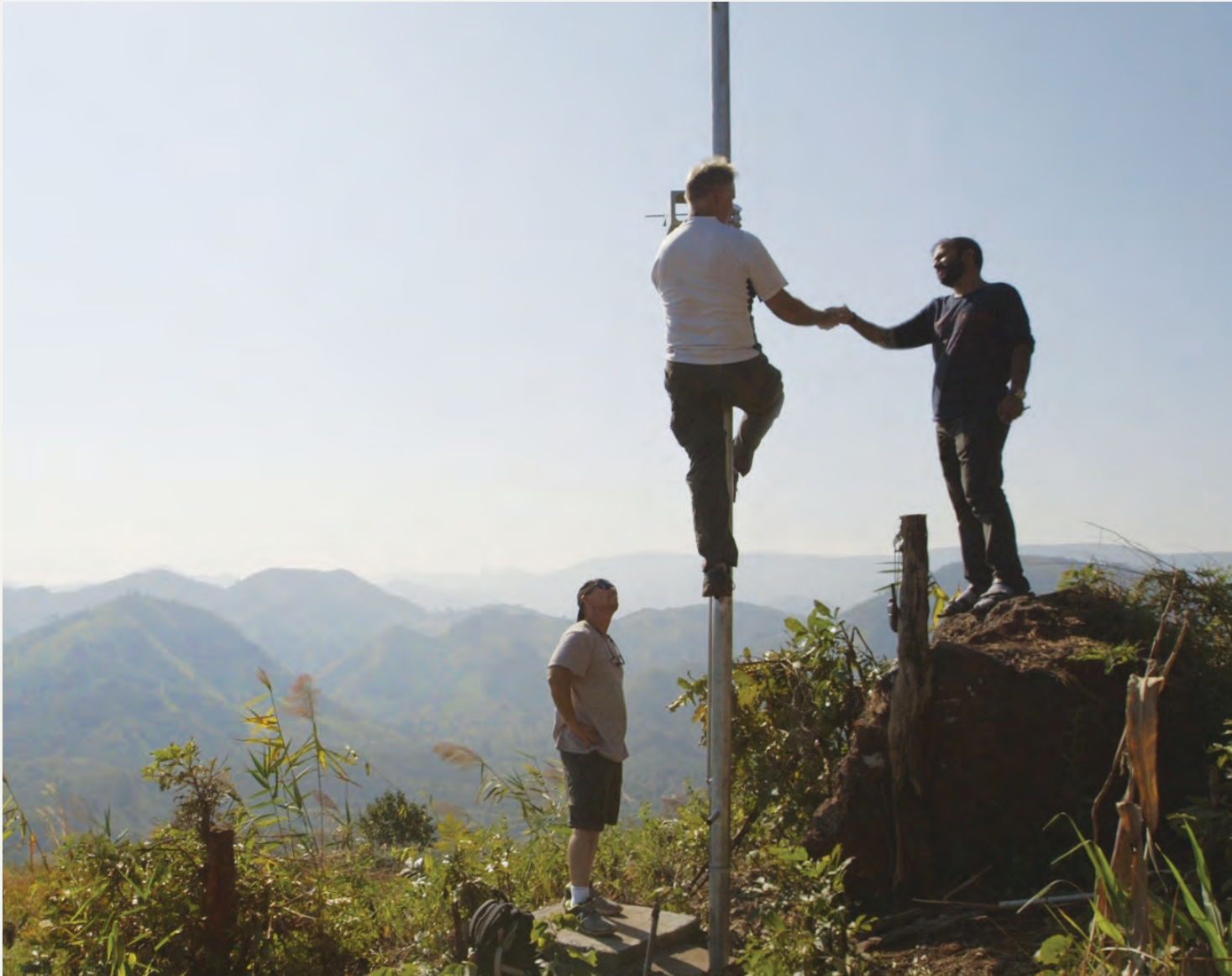
Installing a free space optical communications unit in India
