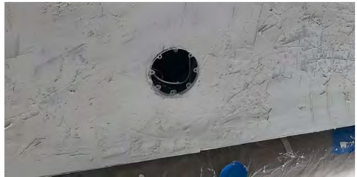
Mounting holes for James Loudspeaker Small Aperture speakers
