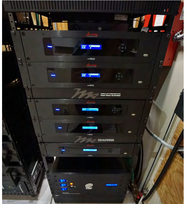
Rack of James Loudspeaker M1000 1000-watt subwoofer amplifiers
