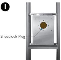
Determine the placement of the Small Aperture sub assembly and secure the unit between two wall studs.We recommend using a block of wood, fixed between the studs, to aid in the leveling process (Wall mounting process shown).
