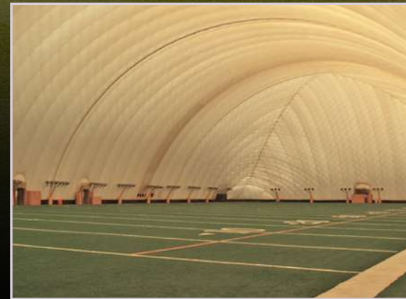
INDOOR PRACTICE FACILITY
