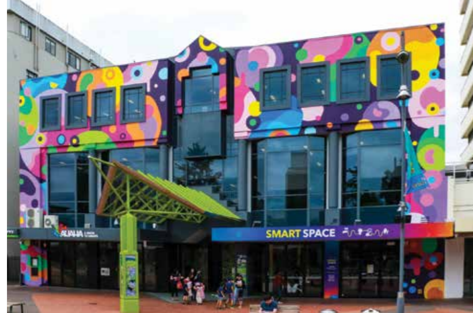
Figure 56: Existing Library in Central City
