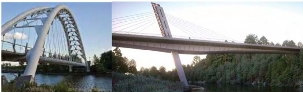
Figure 19: Tied Arch and Cable Stayed Concepts
