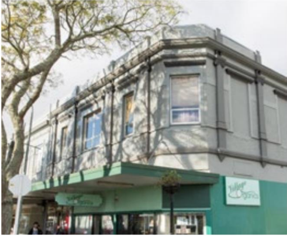
Former Frankton Junction Supply Store - 245 Commerce Street, Frankton. Repairs and painting of building facade.
