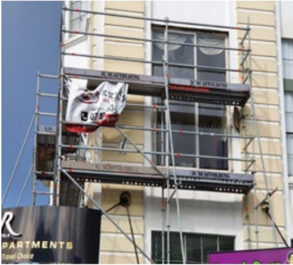
Wesley Chambers - 237 Victoria Street Repairs to the original metal windows.
