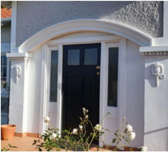
House - 121 Grey Street - Repairs and Maintenance
