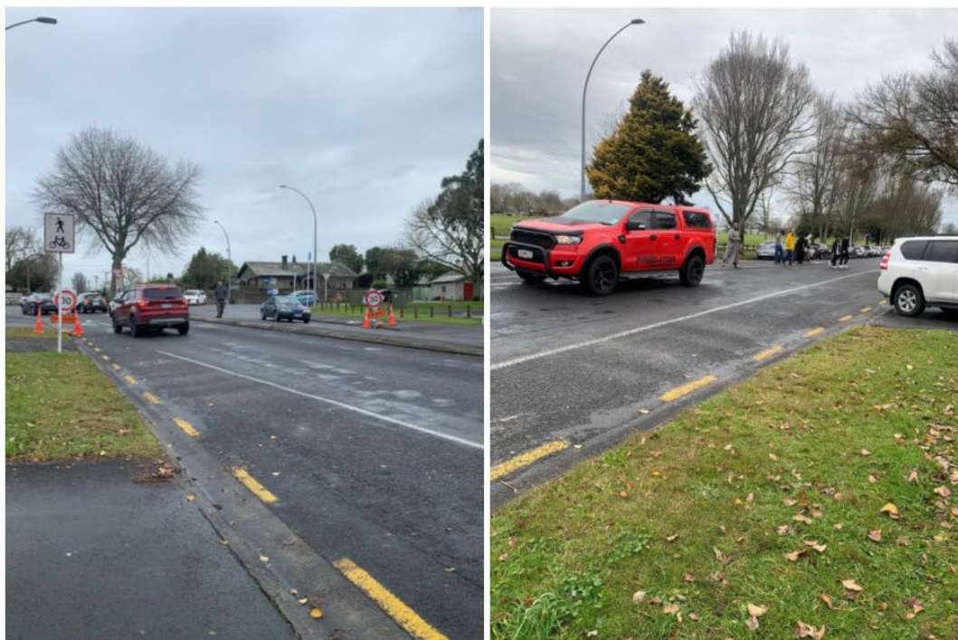
Figure 2: Site observation pictures
