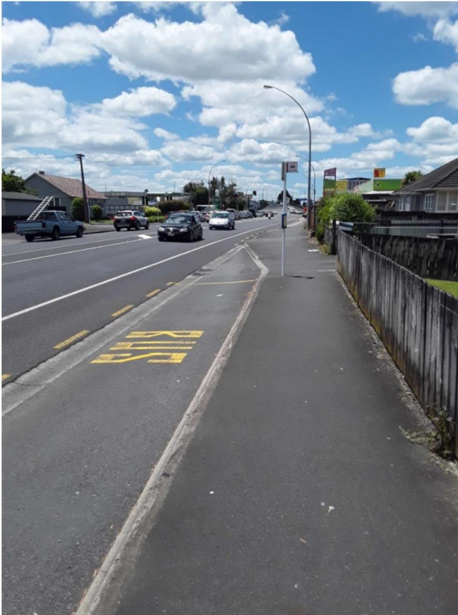
Photo 1 - Indented bus bay with insufficient lead in length, narrow footpath, and kerb damage from buses scraping – Massey Street.
