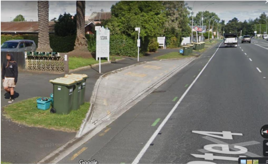
Photo 4 - Indented bus bay with insufficient lead in length, narrow footpath, and steep gradient – Ulster Street near Abbotsford Street.
