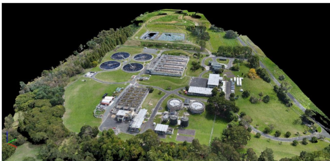
Figure 9: Pukete Wastewater Treatment Plant
